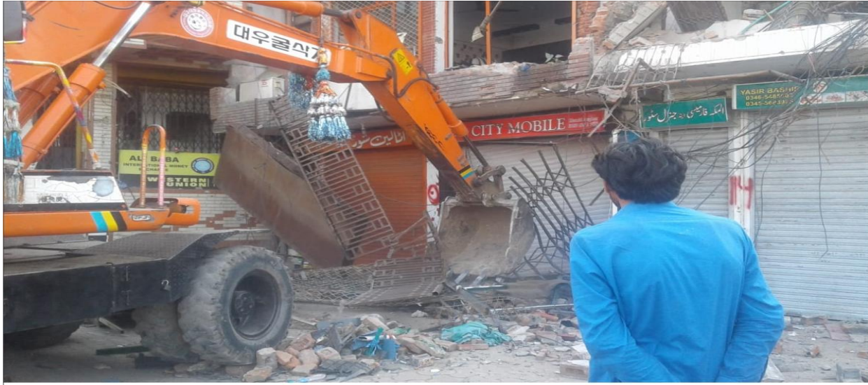
NHA Removing Encroachments from its Right-of-Way
