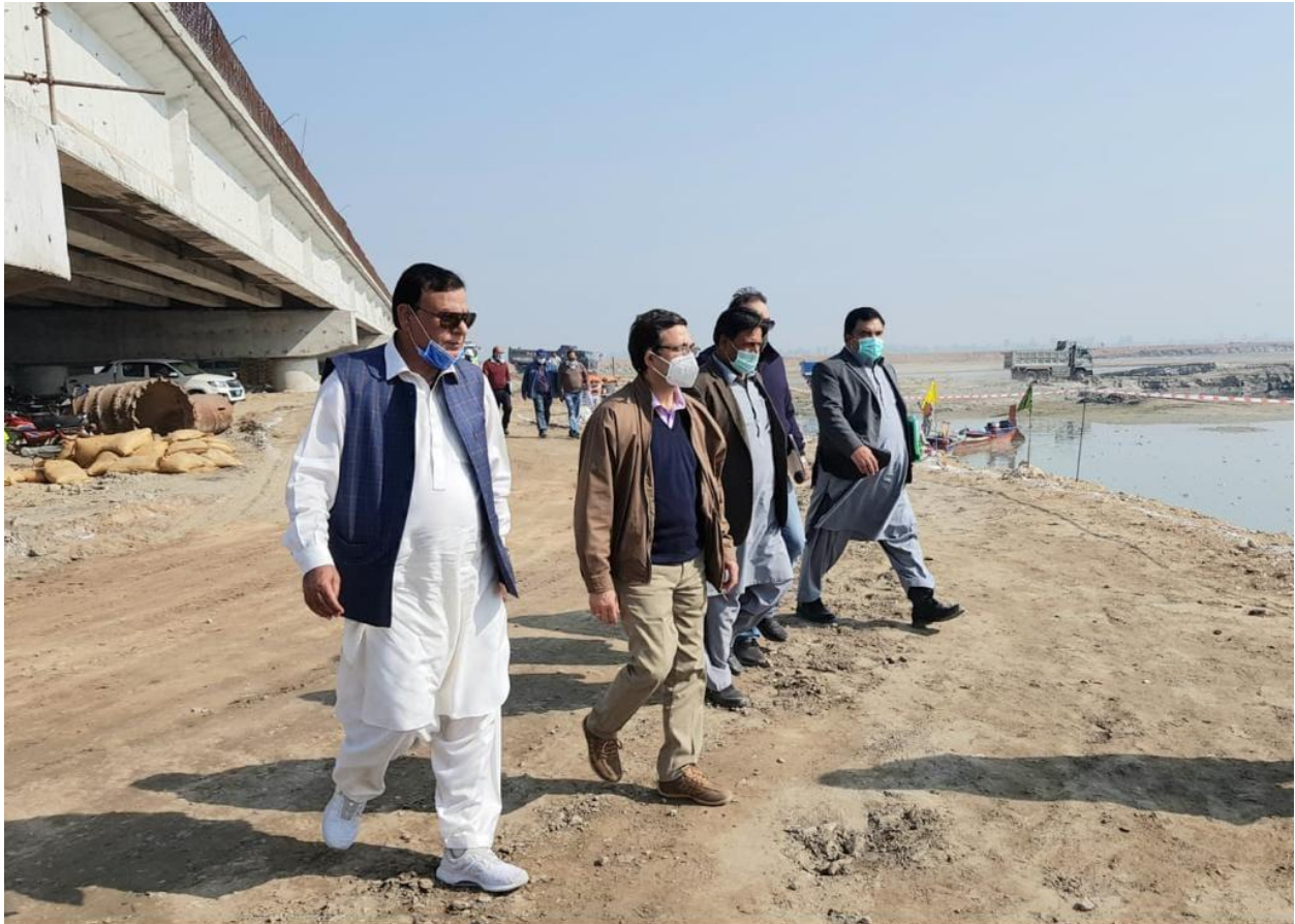
CHAIRMAN NATIONAL HIGHWAY AUTHORITY CAPT ® SIKANDER QAYYUM VISITING UNDER CONSTRUCTION HAKLA - D.I. KHAN MOTORWAY PROJECT (CPEC)
