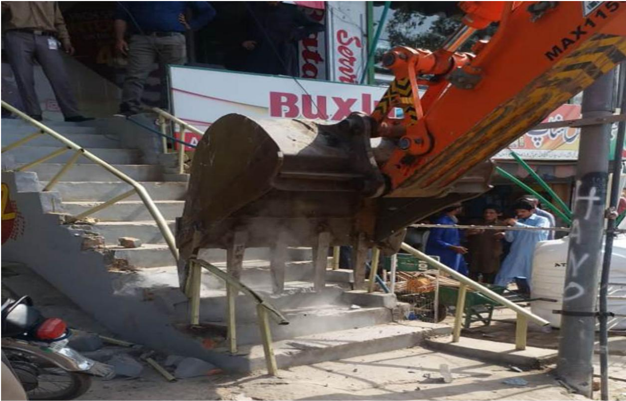
National Highway Authority is removing encroachment from its Right of way.
