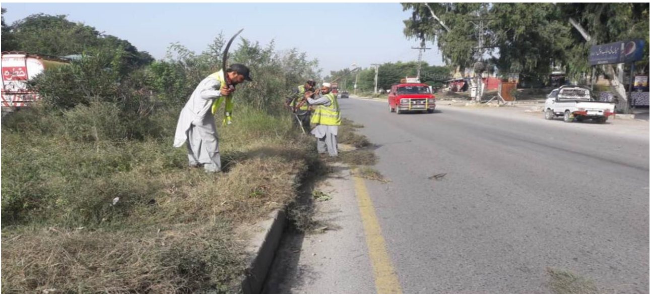
Vegetation cut work along National Highways in progress.
