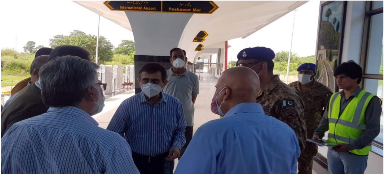
Chairman NHA Capt (R) Sikandar Qayyum inspecting under construction project of Metro Bus from Peshawar More to New Islamabad International Airport.
