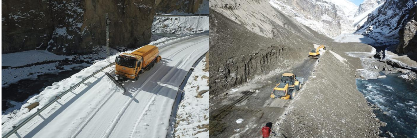
Under auspices of National Highway Authority, snow being removed from Karakoram Highway.
